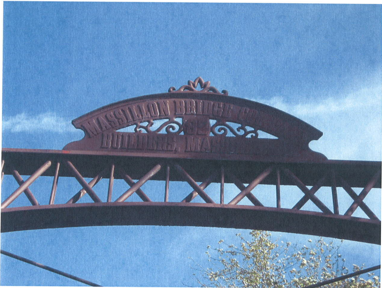
LOG C21-1.00 - NAME PLATE WEST PORTAL
