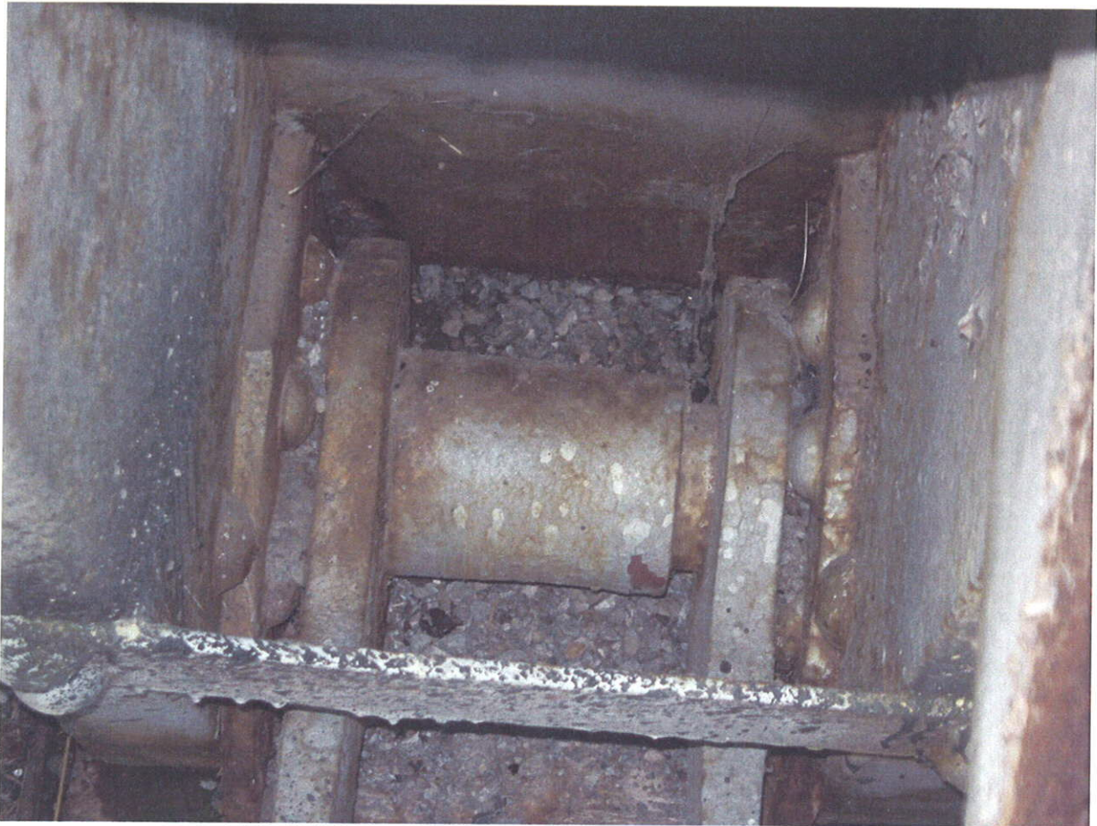
LOG C21-1.00 – TYPICAL BEARING SOUTH WEST CORNER
