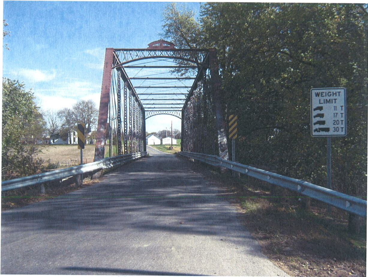
LOG C21-1.00 - PORTAL LOOKING EAST
