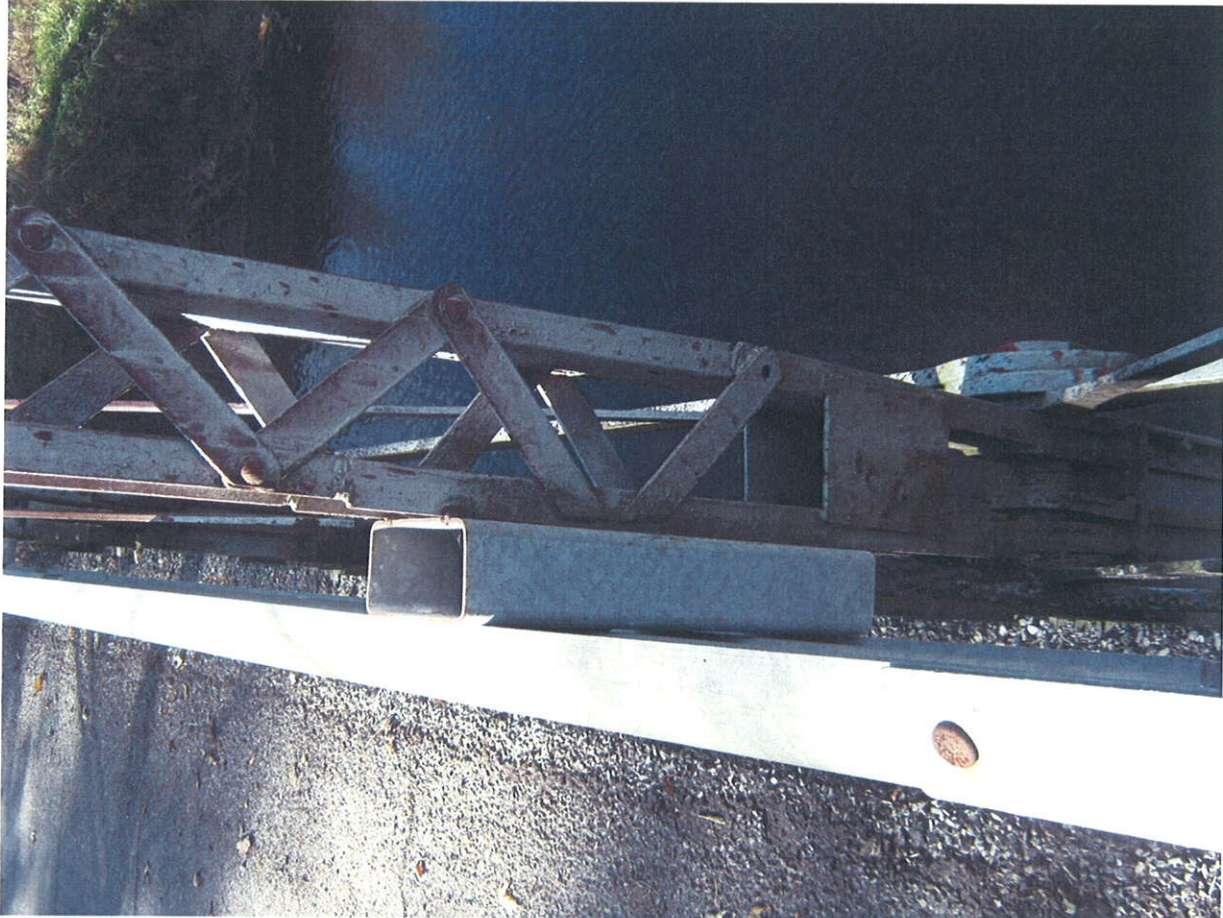
LOG C21-1.00 – EAST SIDE OF U5L5 NORTH TRUSS
