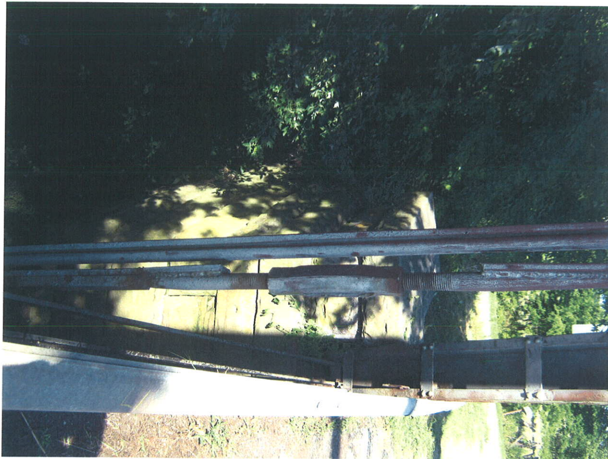
LOG C21-1.00 - L1 TURN BUCKLE REPAIR
