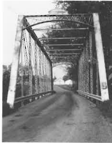
The decorative portal bracing and distinctive nameplate of the Great Miami River Bridge near Logansville are typical of the structures completed in the late 19th century by the Massillon Bridge Company of Massillon, Ohio.
