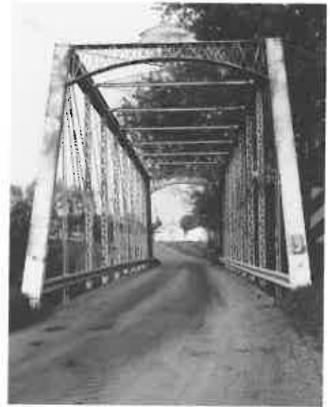
The decorative portal bracing and distinctive nameplate of the Great Miami River Bridge near Logansville are typical of the structures completed in the late 19th century by the Massillon Bridge Company of Massillon, Ohio.
